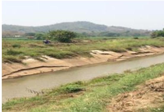
Figure 4. Broken right main canal of the Mae Lao operation and maintenance project
